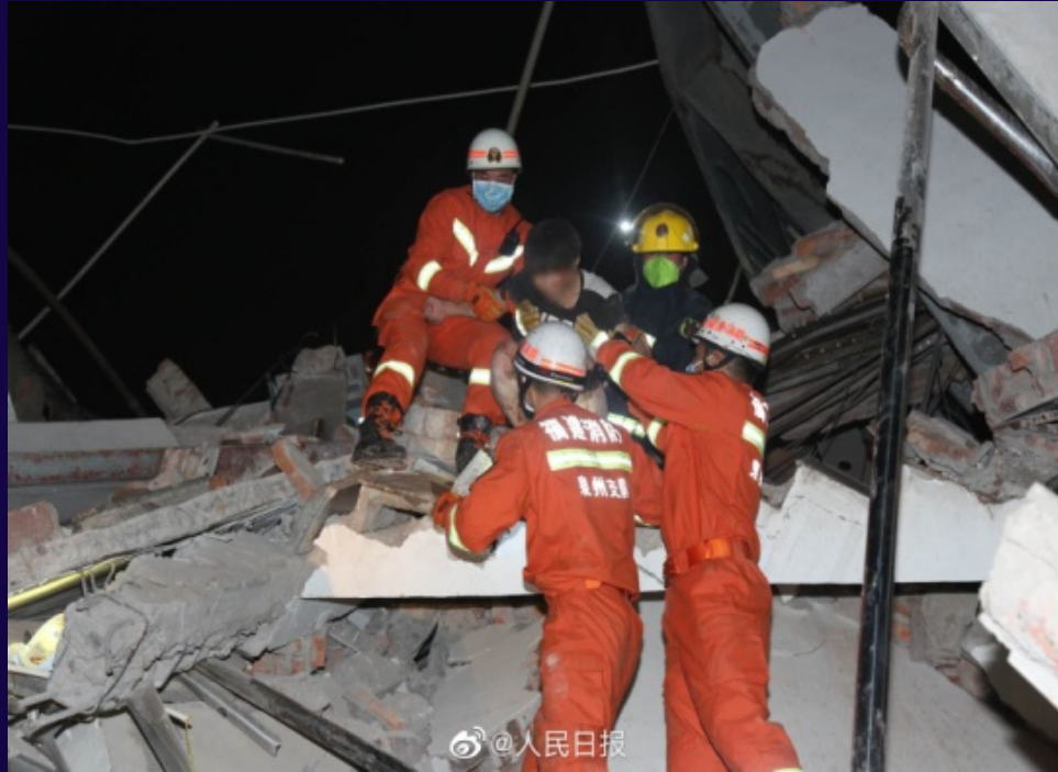
The Xinjia Express Hotel in Quanzhou, China collapsed on 7 March, 2020
